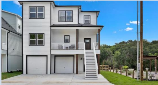
1 st phase of new townhomes at Water Street
