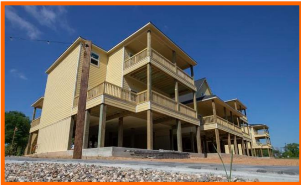
New townhomes underway at Water Street.
