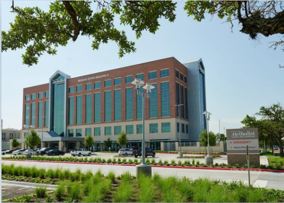
Houston Methodist Clear Lake expansion! New 6-story, 150,000 SF $40M medical office building.
