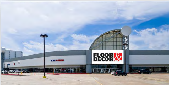
Floor & Décor - 91,000 SF - will open at the Clear Lake Center in Webster, I-45 at FM 528.
