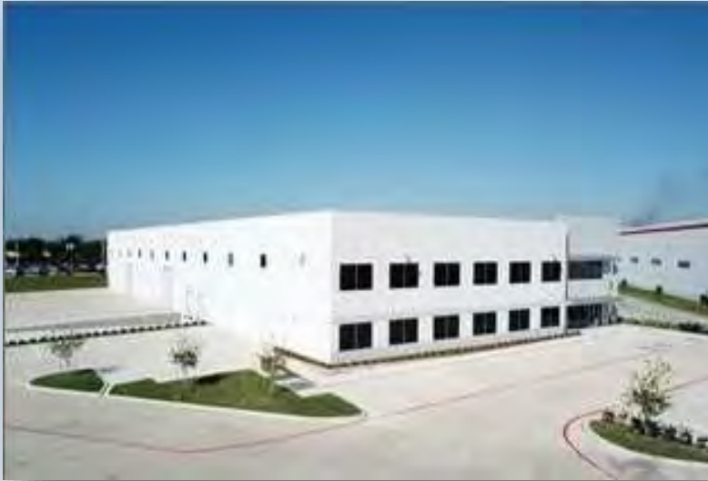
Park 225 - New spec building complete in Pasadena -- 36,954 SF
