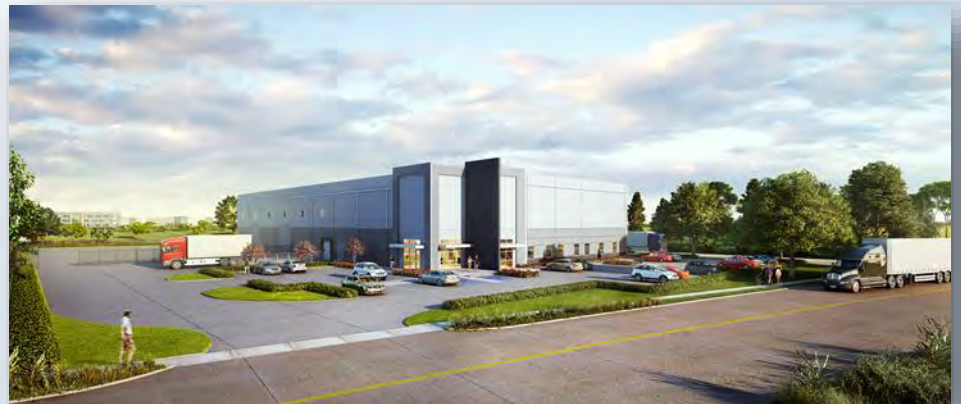
Park 225 at Beltway 8 and SH 225 – Vigavi has underway a BTS for Johnson Controls. 30,000 SF with 7,000 SF office, 40 ton crane capable.
