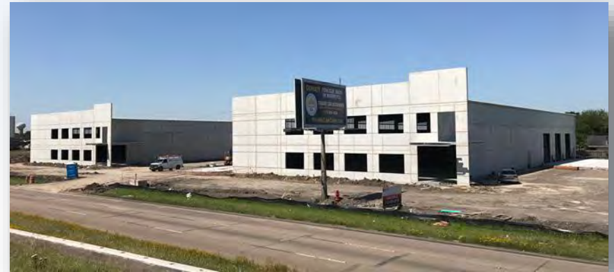
Beltway-225 Business Park by United Equities Inc. Phase II underway – 2 tilt-wall buildings, 22,000 SF and 24,000 SF, both expandable. 30' eave height. Q4 2020 delivery.
